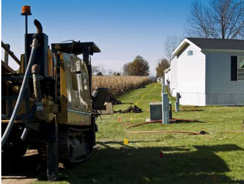
Installation of the fiber backbone and
